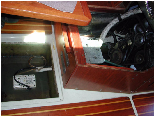
The bilge pump had stopped working.
